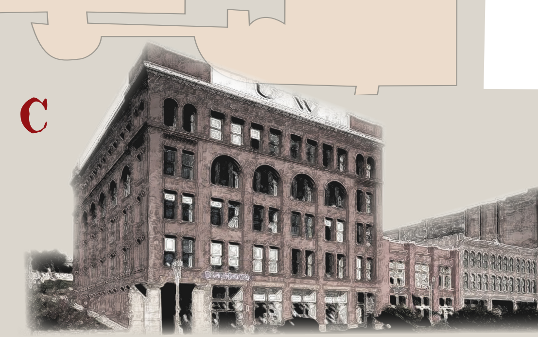
C Garretson Woodruff & Pratt - Built 1891 / Renovated 1995 The optimism and excitement of the economic boom of the late 1880s and early 1900s is reflected in this building, designed by Frederick A. Saxton. Built in a Romanesque style with obsidian pressed brick and terra-cotta trim, the detailing is some of the best in the district. When it was new, a grand staircase offered views of Mount Rainier from the landings.
