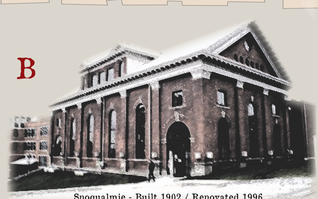
B Snoqualmie - Built 1902 / Renovated 1996 Harnessing the power of the 270-foot Snoqualmie Falls, the Pacific Northwest's first hydroelectric plant began producing electricity for Tacoma and Seattle in 1899. This building, erected a few years later, housed the giant transformers needed to reduce the voltage coming directly from the plant. The Snoqualmie Falls Power House supplied electricity to most of Tacoma, including the 600 volts needed for the electric trolleys.
