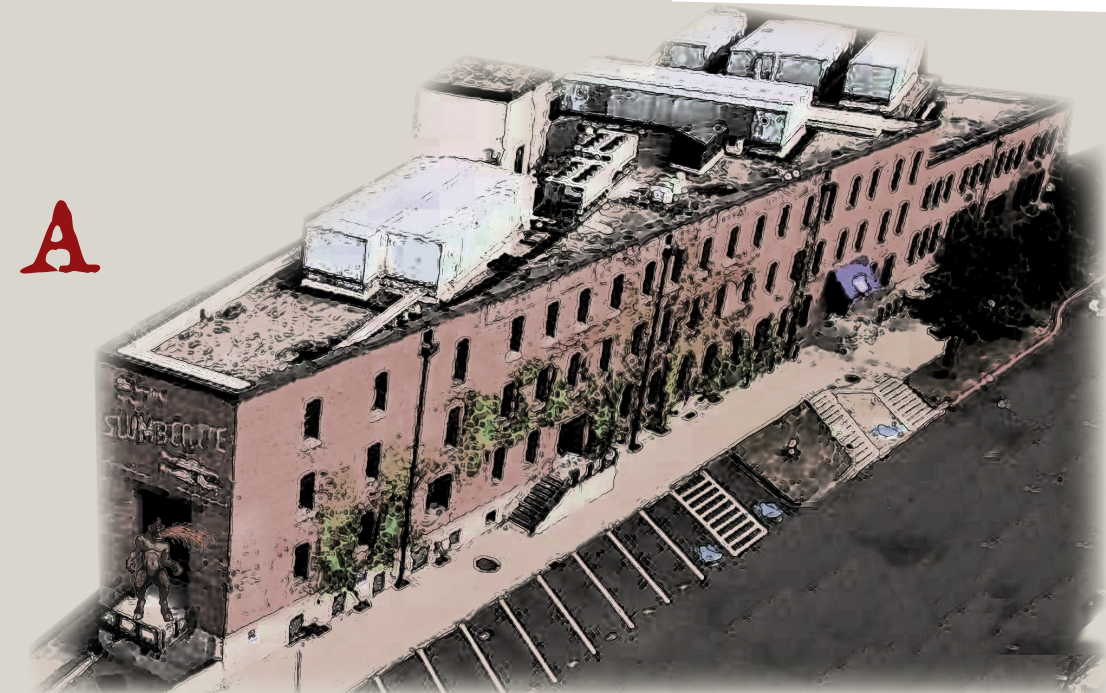
A The Mattress Factory - Built 1908, 1912 / Renovated 2003 The Mattress Factory is made up of two buildings with very different histories. The southern part was originally the Lindstrom-Berg Cabinet Works and the northern part was a factory built for the Harmon Furniture Company. "Ghost writing" ads for the firm can still be seen on the building's exterior and on other restored buildings on campus.
